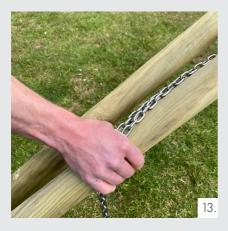
Now carefully separate the poles to create a sturdy tripod. Make sure the DIY-base is positioned as horizontally as possible. See photo 14
