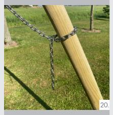
3. When, after a while, the chain runs stiffly over the guide, a little (vegetable) oil can work wonders. Put a drop of oil on the tube that the chain is running over and pull the chain over it a few times. The chain will run more smoothly.
