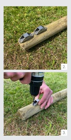
The hinges can now be fixed to the posts with 1 wood screw per hinge. Repeat this for all 3 posts. Make sure that the hinges are reasonably tight on the wood but can still move. See photo 4
